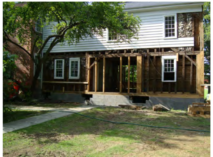
Southworth house, steel beams removed and ready to complete the foundation
