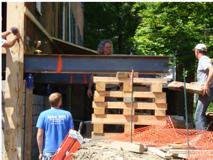
Contractor, Mike Walker begins removing cribbing supporting steel beams
