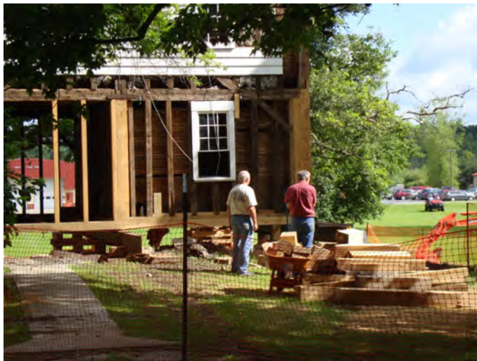
Southworth House up on steel beams - Albert Heidt, Bob Watros
